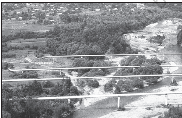
Fig. 8.17: Pipelines transporting natural gas in Ukraine
